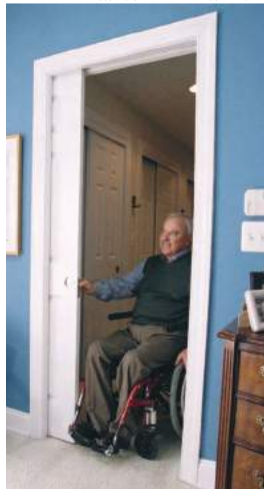
Pocket doors do not require as much maneuvering space as swinging doors, but the adjacent wall space must be wide enough to accommodate the door and be clear of utilities and structural parts.
