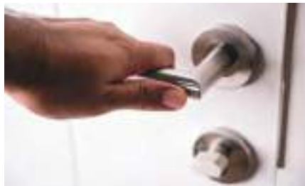
Lever-style lockset hardware should be used on all doors to ease use for those with limited hand dexterity.
