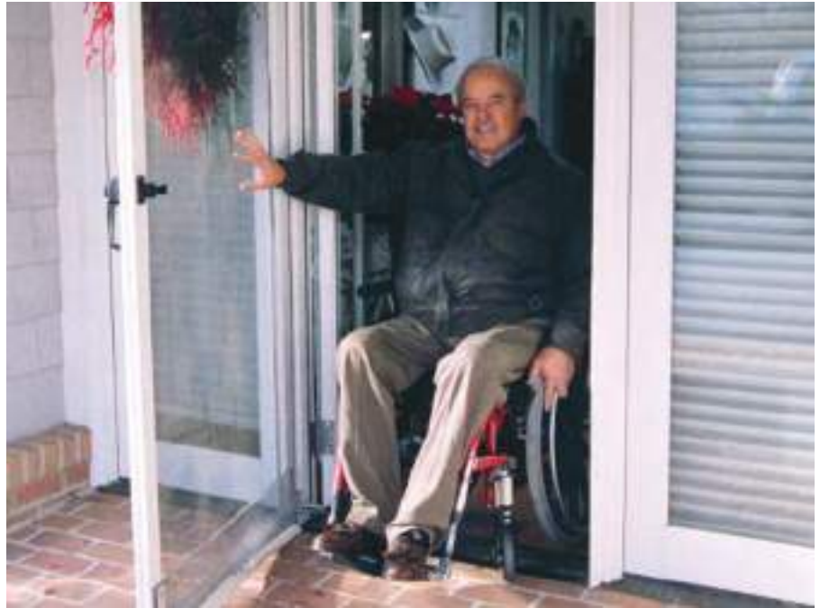
A low-profile exterior threshold along with a gentle exterior slope away from the door combines a good weather barrier with relatively level transition from inside to out. The storm door is protected along its bottom by a kickplate accessory. For safety, glass sidelights provide exterior visibility.
