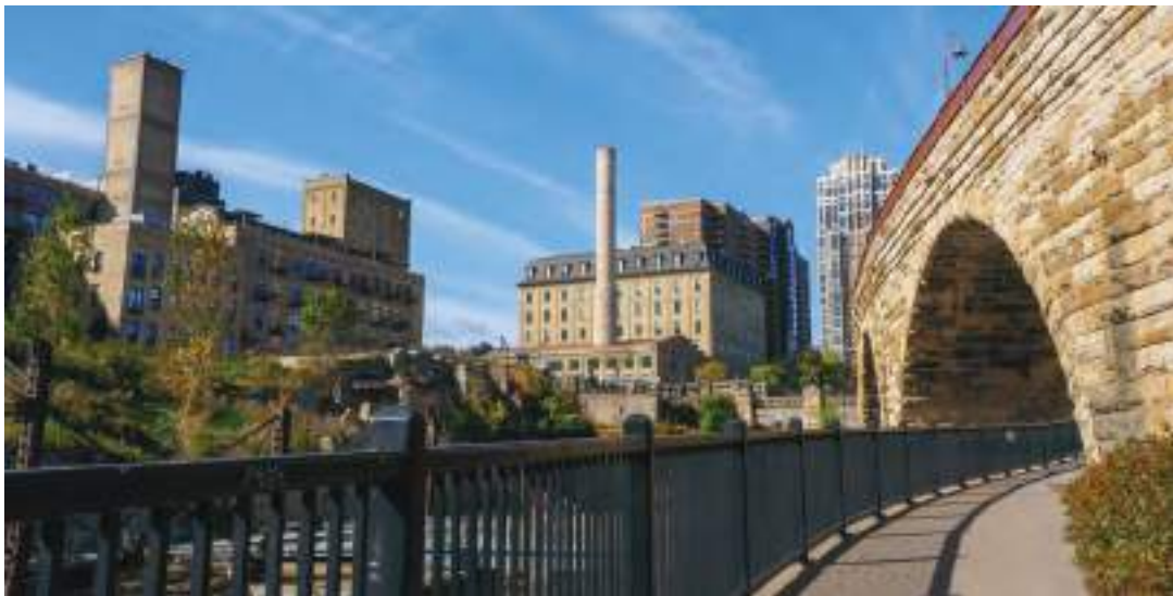
Mill Ruins Park features the Stone Arch pedestrian and bicycle bridge.
